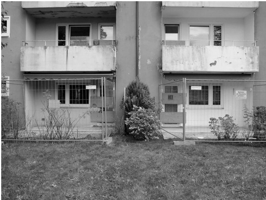
AHA wins balcony repairs, © Photo: AHA Munich
